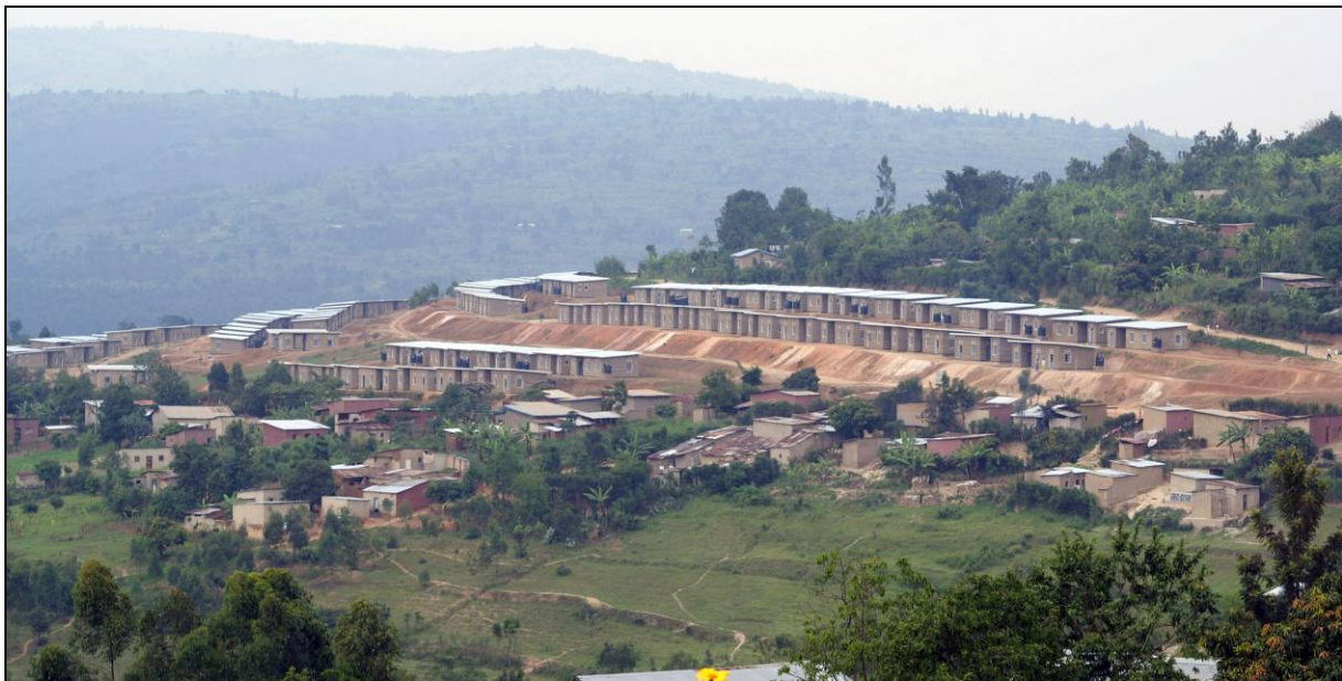
Photo 4 - Batsinda pilot community under construction, February 2008 (1°54'2.29"S, 30°4'36.61"E).
