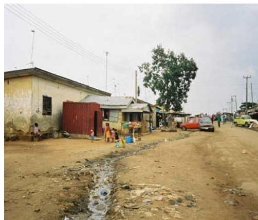
Figure 4. A road in Nyanya showing blocked drainage sources ( no bins)
