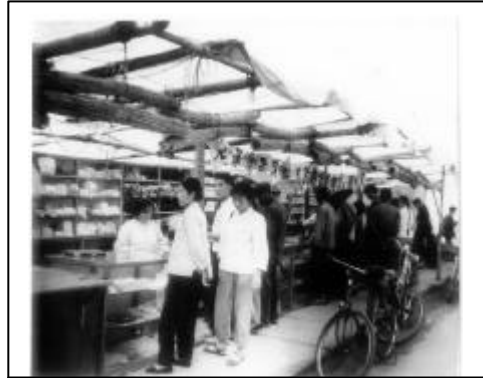
Transitional market after earthquake
